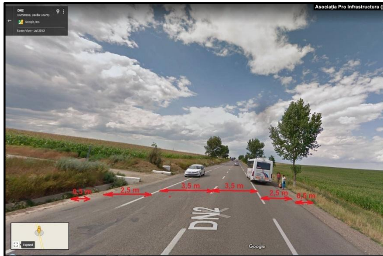
Figure 17. National Road 2 (DN2), which from a construction point of view does not offer road traffic safety due to undersizing [12].
