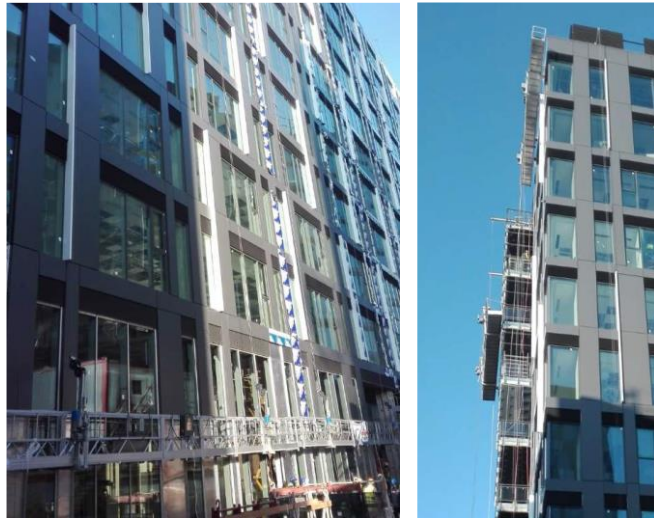
Figure no. 1 - Images of Bridge III site platforms
