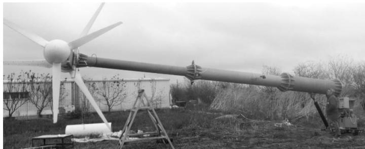
**Figure 11.** Hydraulic prop- wind turbine lifting by mobile pumping, distribution and control unit.
